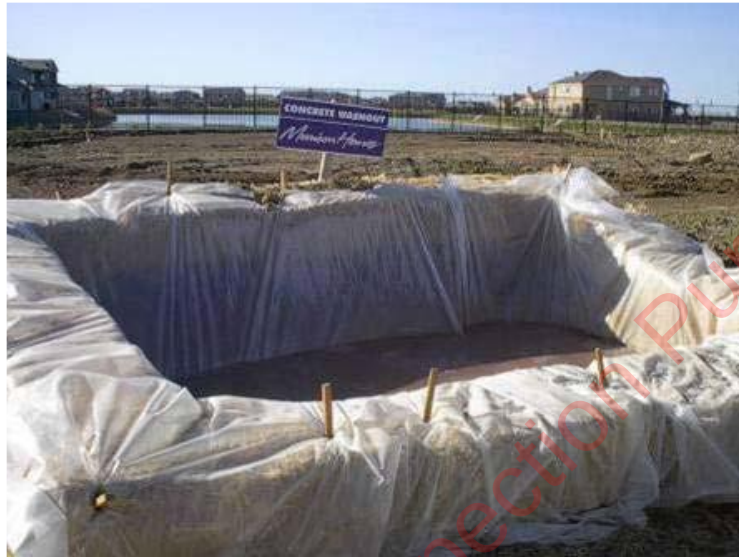
Plate 2.1: Typical Temporary Concrete Washout Area
